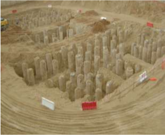
Pile cap excavation in progress (Oct-08)
