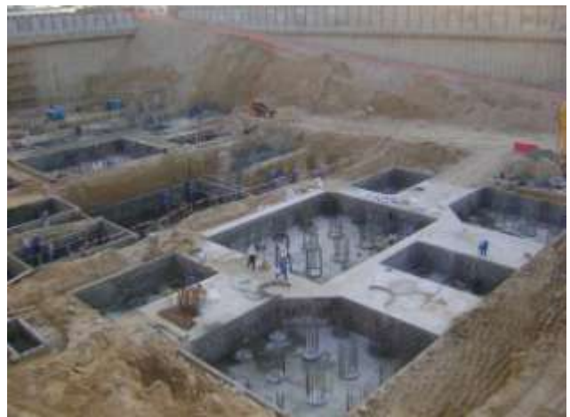
Raft works in progress Tower B (Dec-08)
