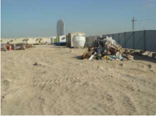
Site before excavation (Nov-07)
