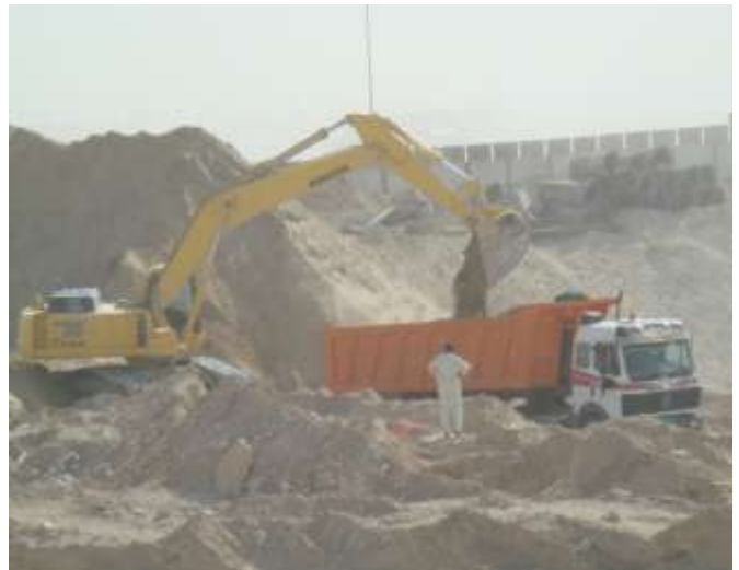
Excavation, Transportation in progress (Jul-08)
