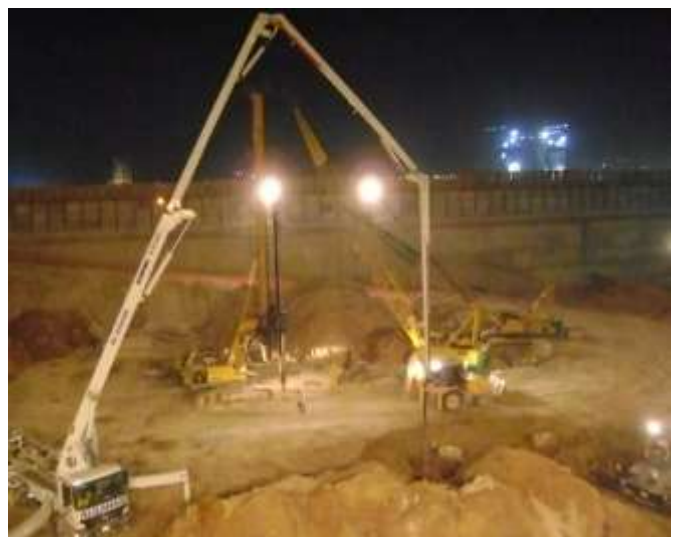
Concreting of piles in progress (Sep-08)
