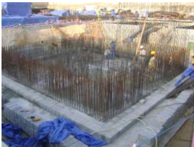
Steelwork for lift wall in progress (Jan-09)
