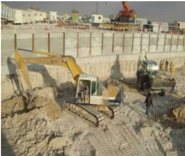
General excavation in progress (Apr-08)
