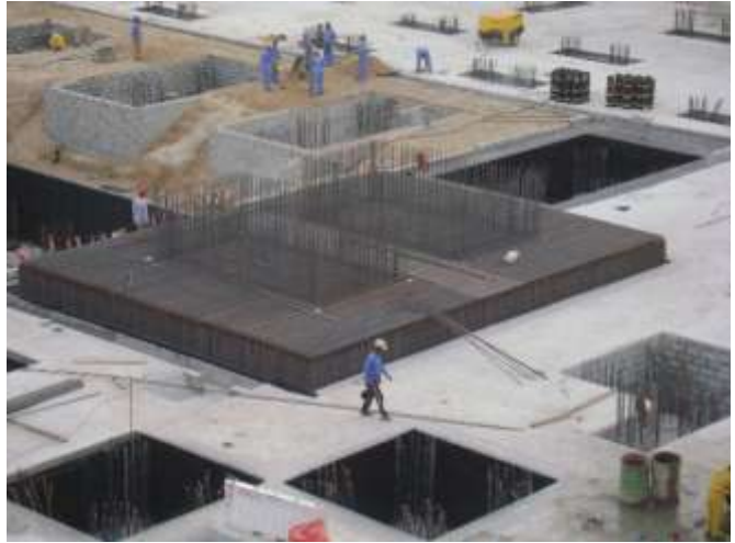
Reinforcement works in progress (Dec-08)
