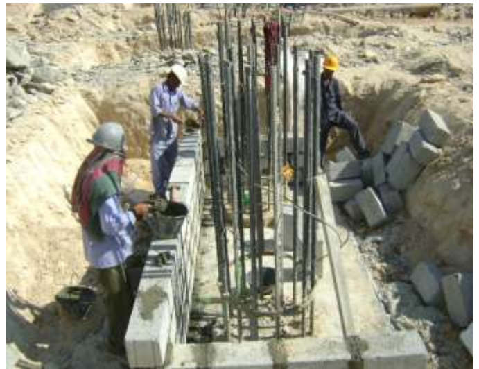
Block work for pile cap in progress (Nov-08)
