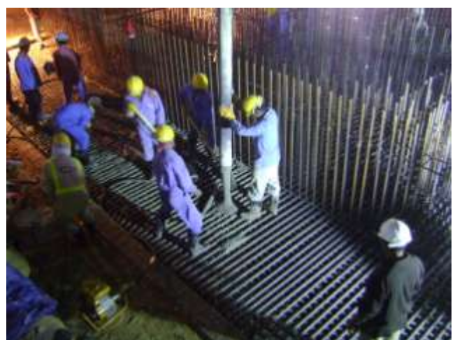
Concreting for lift wall in progress (Jan-09)
