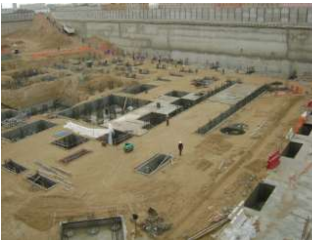
Raft work in progress Tower A (Nov-08)
