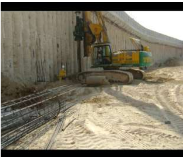
Boring of piles in progress (Aug-08)
