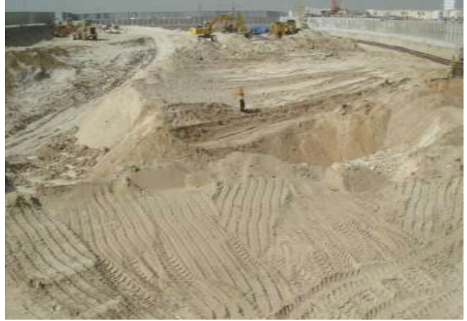
Site after fencing and shoring (Feb-08)
