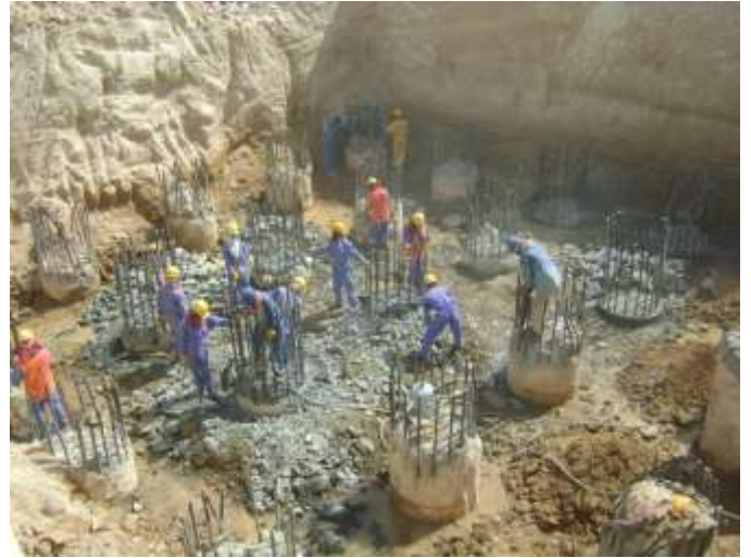
Pile head breaking in progress (Oct-08)
