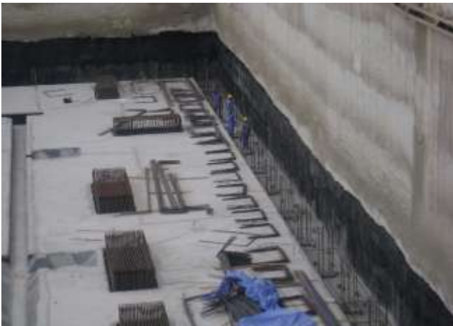
Retaining wall steel work in progress (Dec-08)
