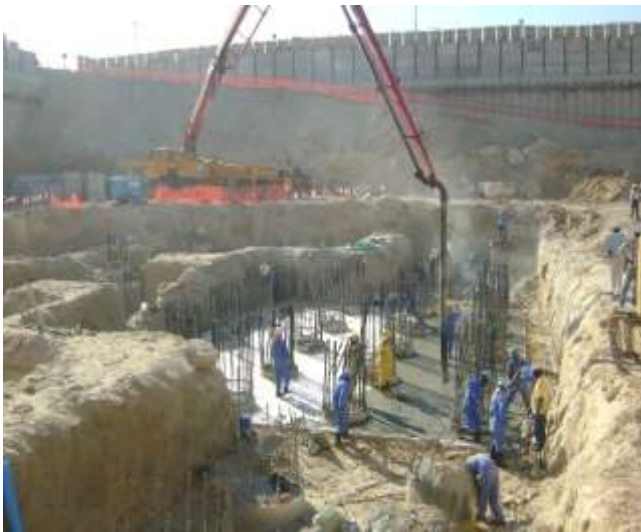
Blinding for pile cap in progress (Nov-08)
