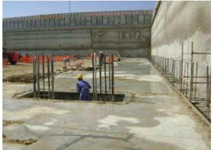
Blinding of raft in progress (Nov-08)
