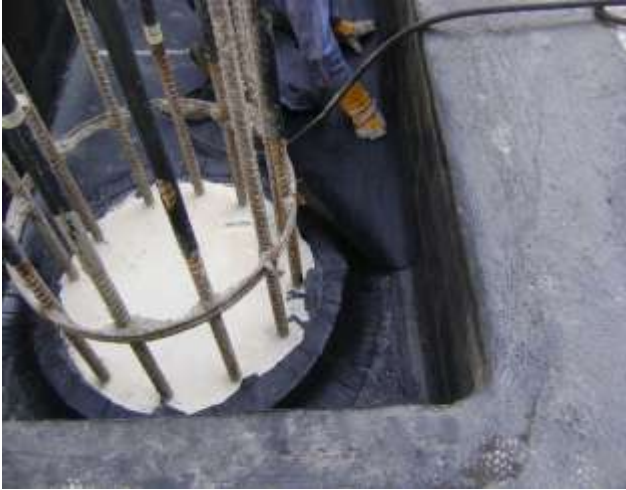
Waterproofing works in progress (Dec-08)
